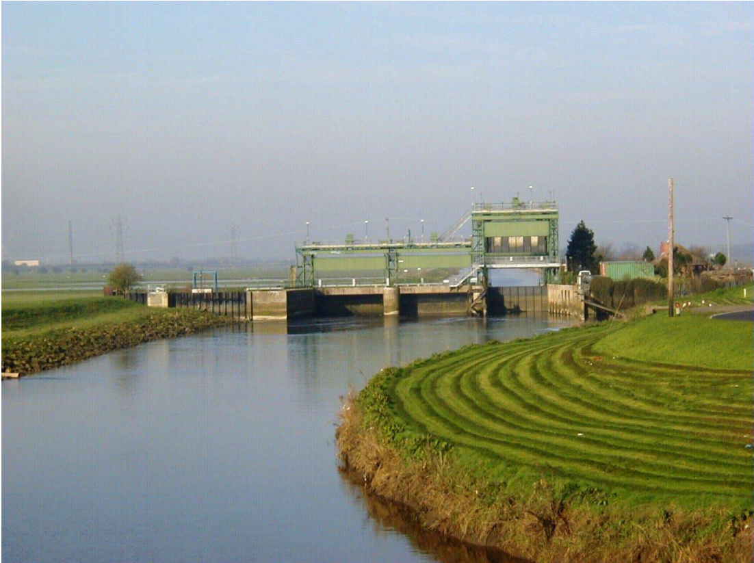
Figure 7-3: Dog in the Doublet sluice when the tide is not so high. Source: Environment Agency.
