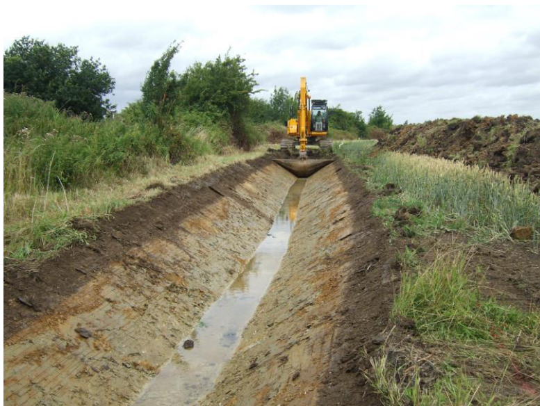
Figure 10-1: Completed action to create a new ditch near Eye Green to reduce flooding
