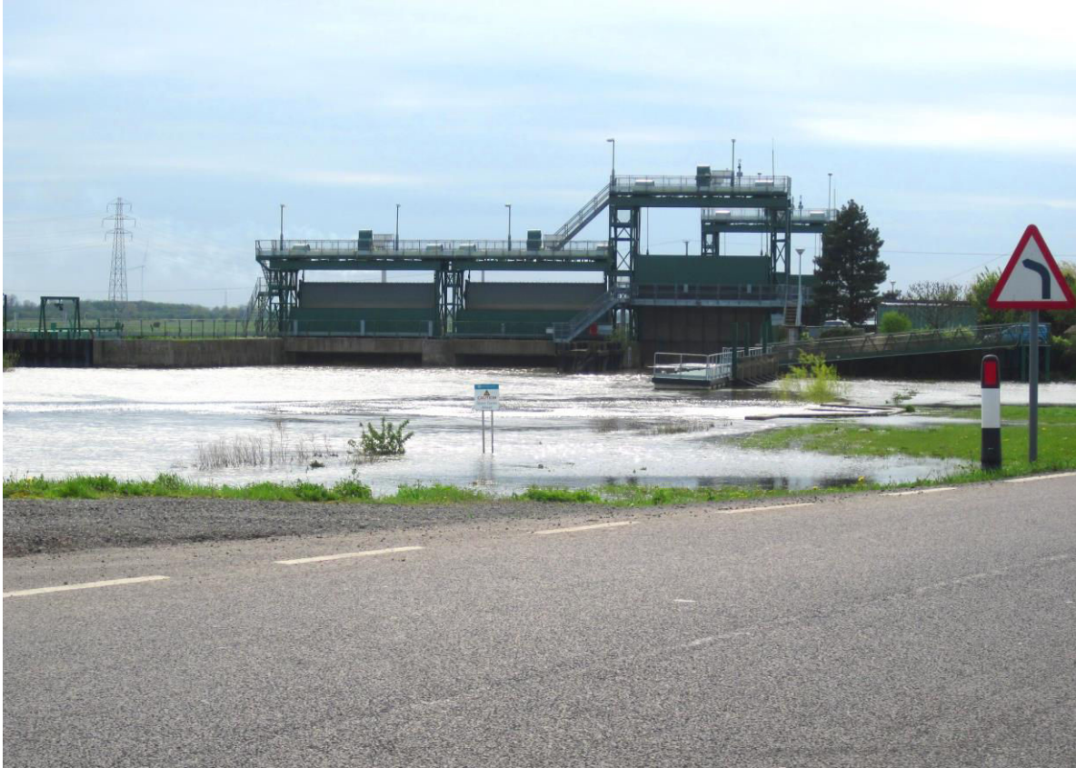
Figure 7-2: Dog in the Doublet sluice during a very high tide. Source: Peterborough City Council
